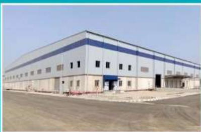
Ware House Construction
