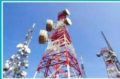
Electrical Work & Telecom Towers
