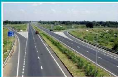
Expressway Road Works
